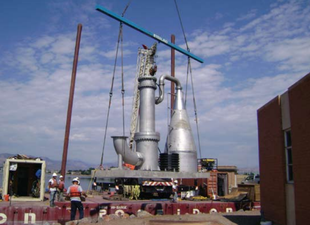
Figure 4. Loading the Speece Cone on to the barge prior to installation.
