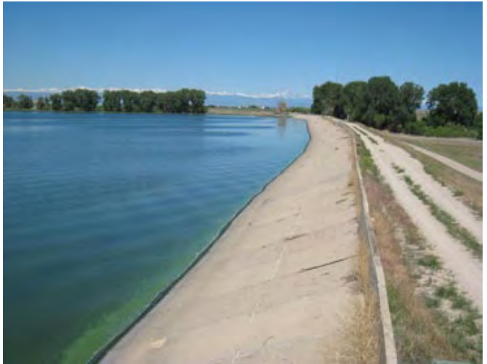
Barr Lake Dam
